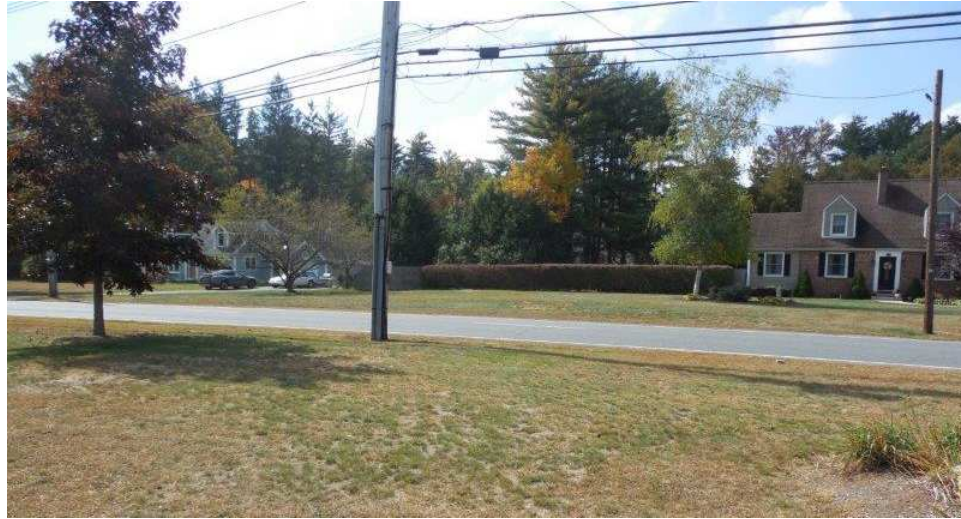
utility pole on Allen Street
