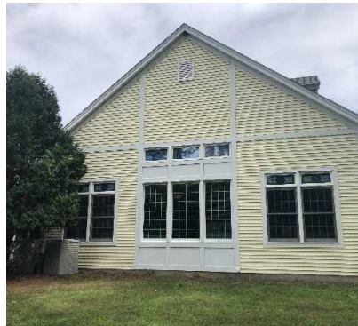
exterior view of windows
