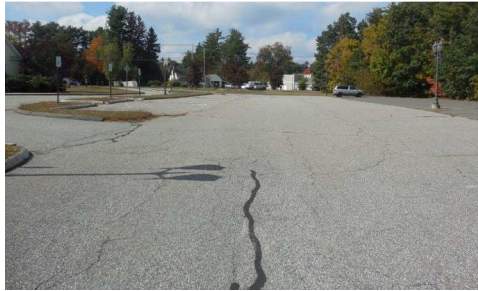
cracking pavement
