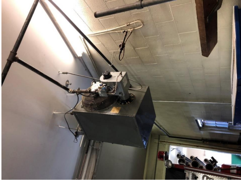
M-3 Gas Fired Unit Heater
