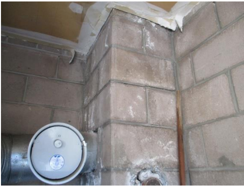
03 – Ceiling and Chimney in Mech. Room
