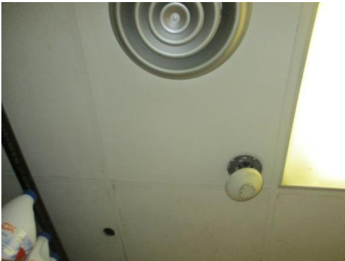
01 – Old ceiling assembly and hanging detector
