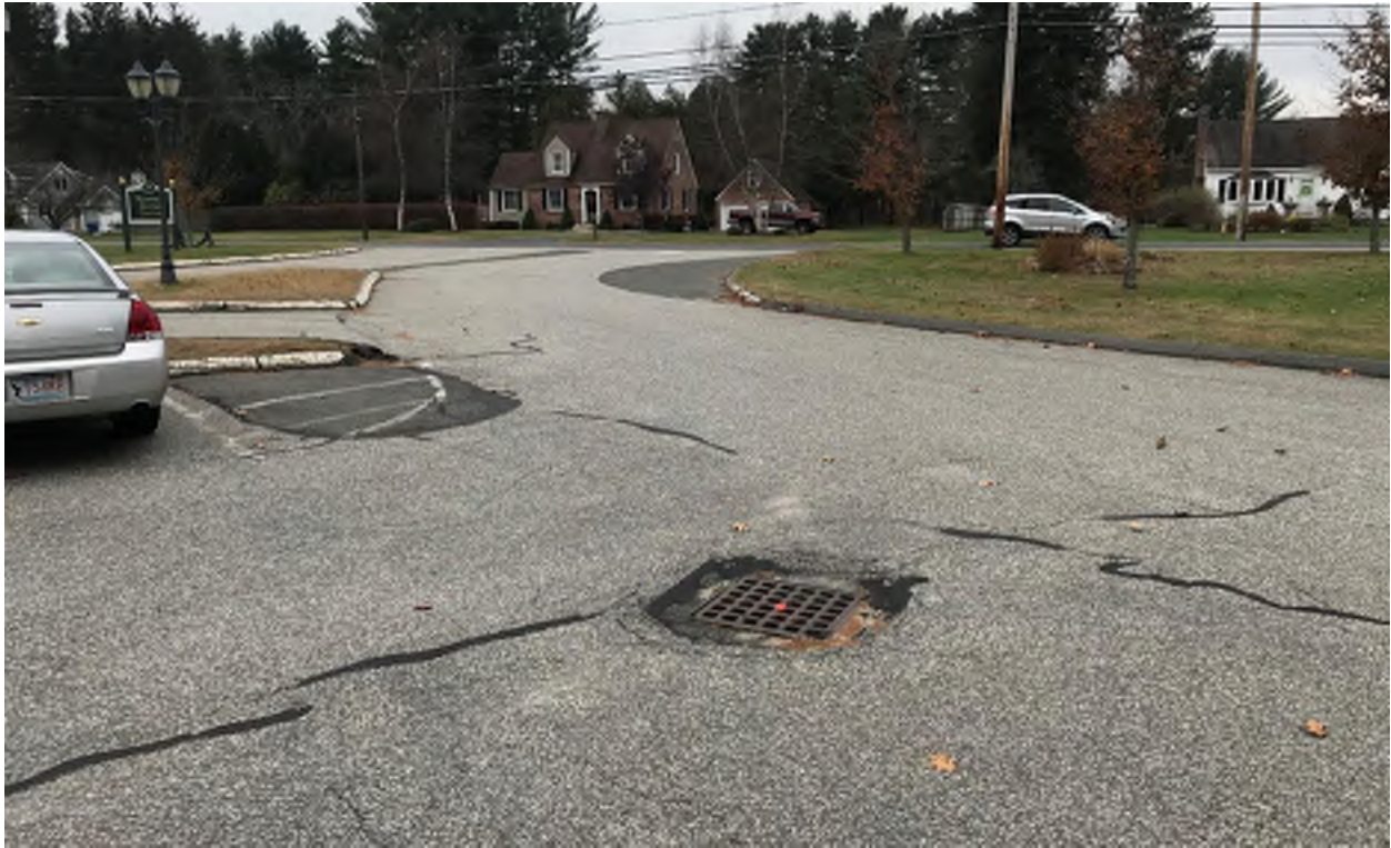
Photo 49. Catch basin in the parking area of the Hampden Senior Center, looking south toward Allen Street (November 7, 2019). The three catch basins at the Senior Center are leaching basins.
