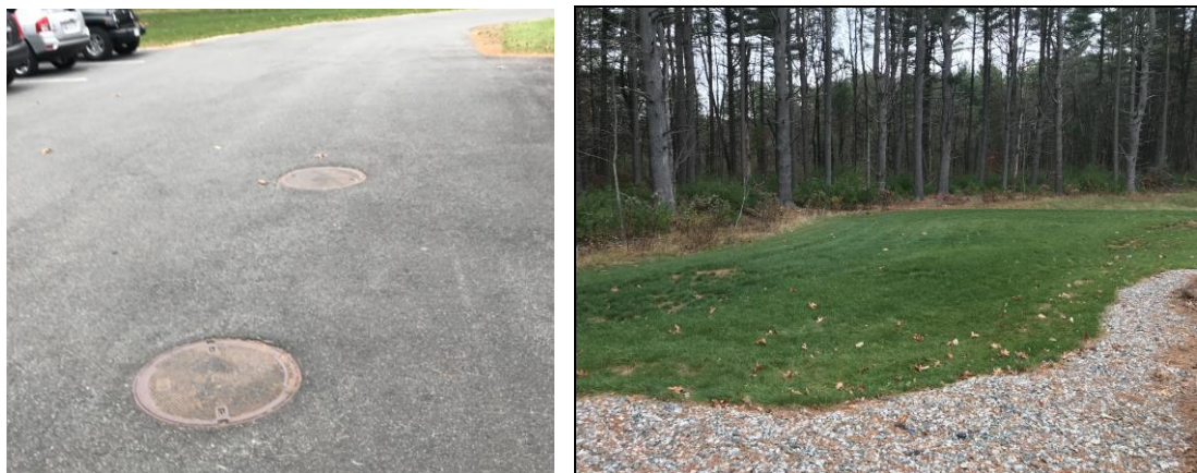
Figure 3.2.: Manholes for the double-chambered tight tank (left) and on-site wastewater treatment system leachfield (right) at the Hampden Police Station.
