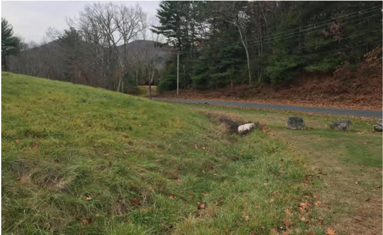
Photo 33. Swale at the base of the capped landfill of the Transfer Station and Recycling Center, looking southwest toward Cross Road (November 7, 2019).
