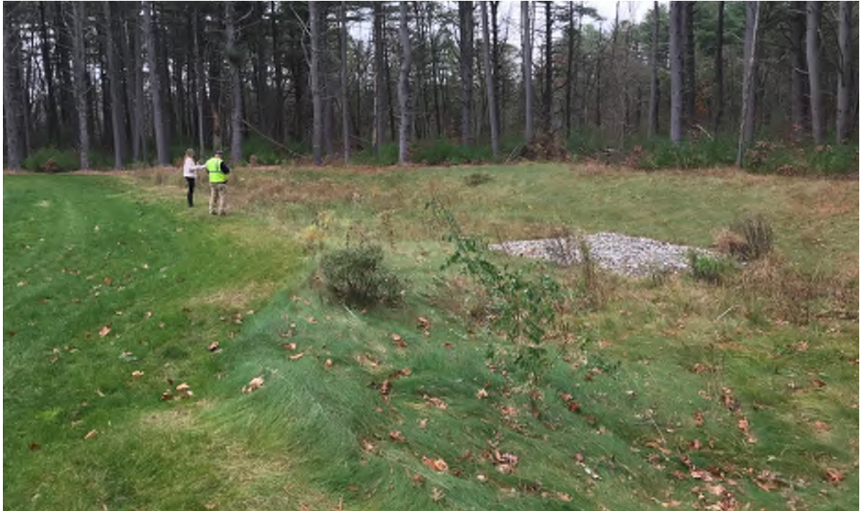
Photo 55. Retention basin located on the southeast side of the Police Station parcel. There are no visible inlets, the site appears to be graded for sheet flow to the basin (November 7, 2019).
