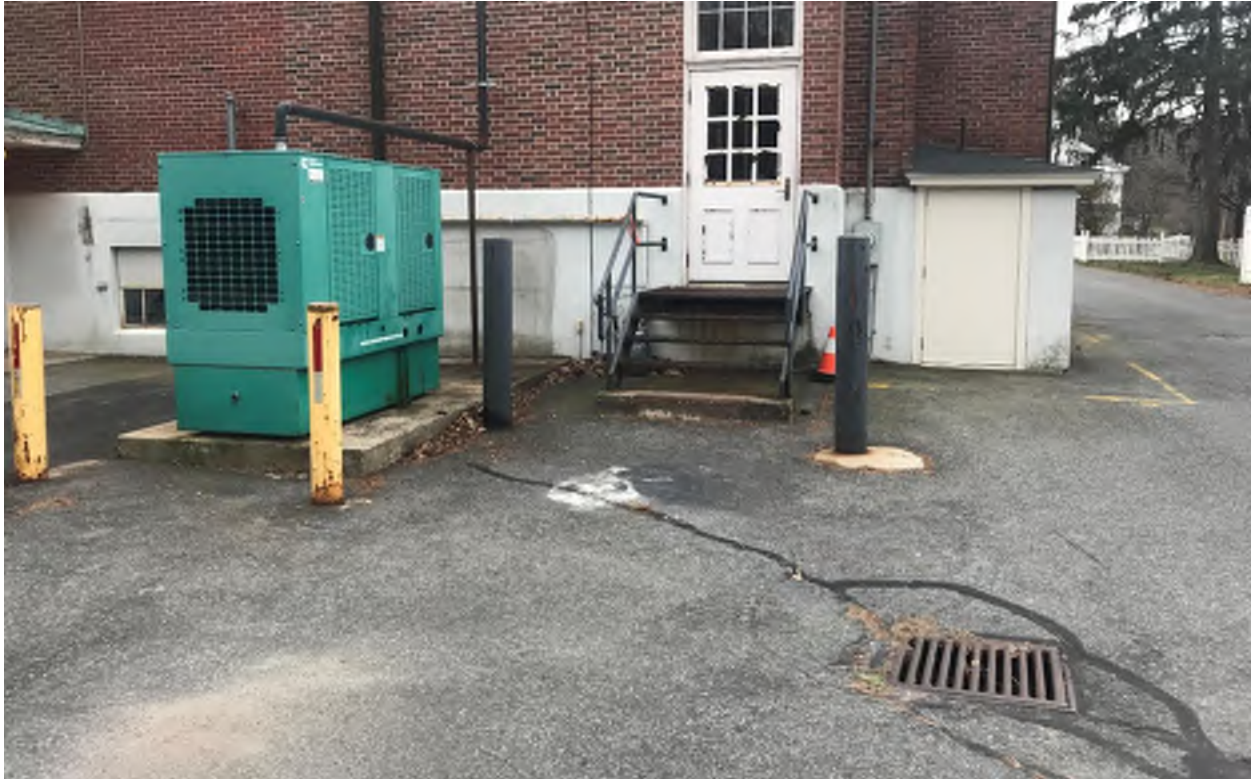
Photo 23. Looking south at the catch basin in the parking area of the Hampden Town Hall/Library (November 7, 2019). The roof drains in this part of the building are connected to the catch basin.
