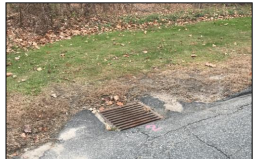
Figure 6.1. Labeled catch basin off of the Highway Garage driveway.
